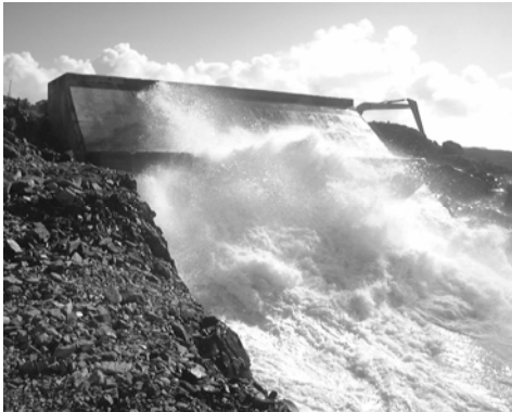
Figure 14-2 Shoreline OWC – the LIMPET
