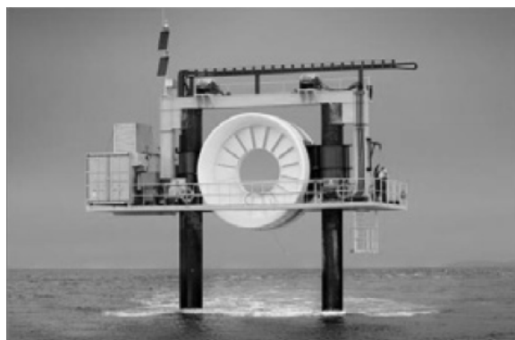
Figure 13-9 The OpenHydro system installed at EMEC Source: OpenHydro
