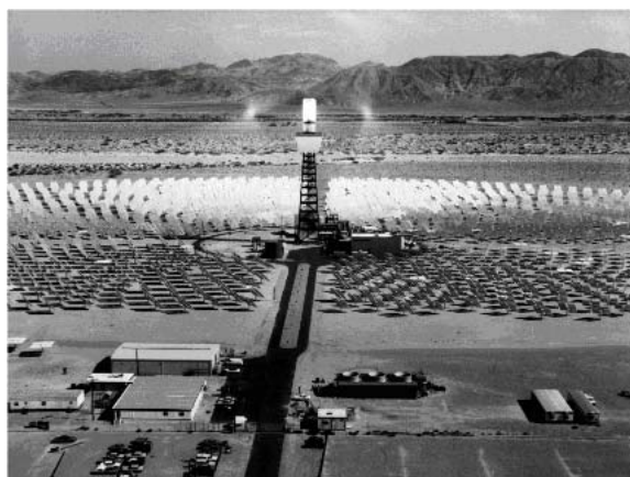
Figure 10-16 Central receiver power plant in California Source: Goswami
